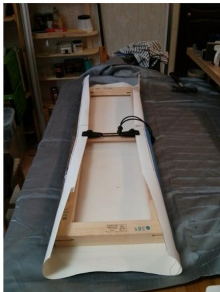
Additional straps are fixed at regular intervals and the alignment checked again before fully tightening.
